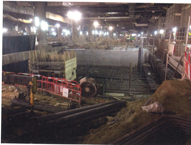
Image 1: Bottom layer rebars in Area C1 of EWL slab (West)
