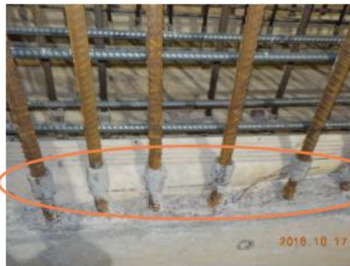
Box 219 - Couplers at Trough Walls
