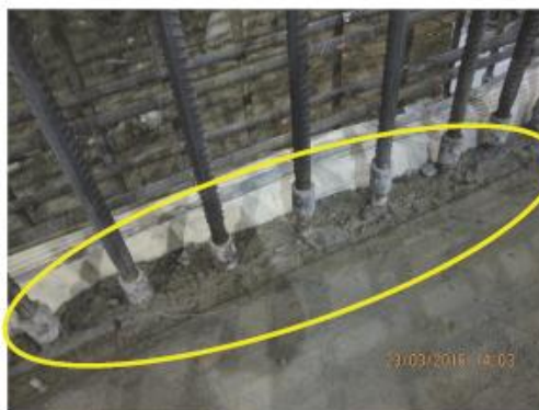
Box 284 - Couplers at trough wall
