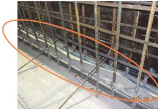
Box 108 - Couplers at Trough Walls
