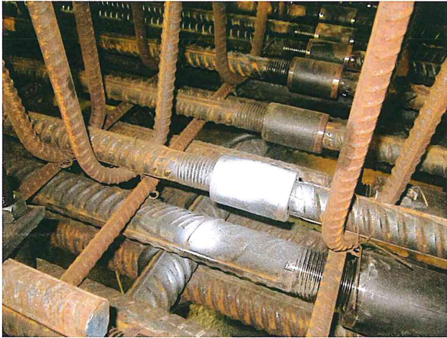
Image 8: inspection of coupler connections during trial in July 2013
