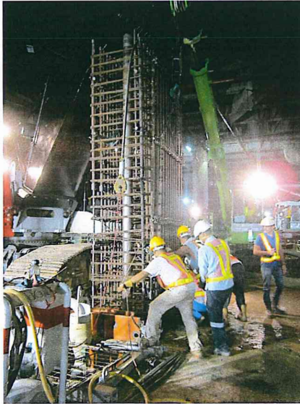
Image 14: splicing works at location of panel EM 98
