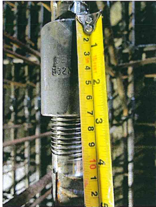
Image 16: measurement of exposed thread
