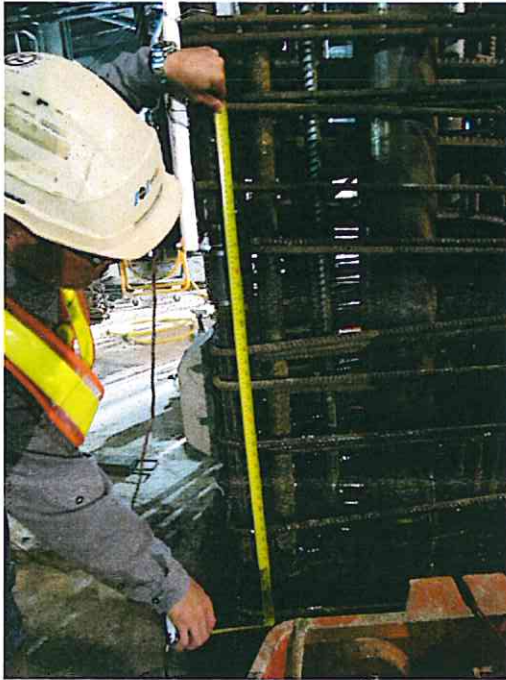
Image 15: splicing of 2 nd and 3 rd steel cages
