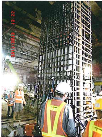
Image 12: rebar cages being installed at location of panel EM 98
