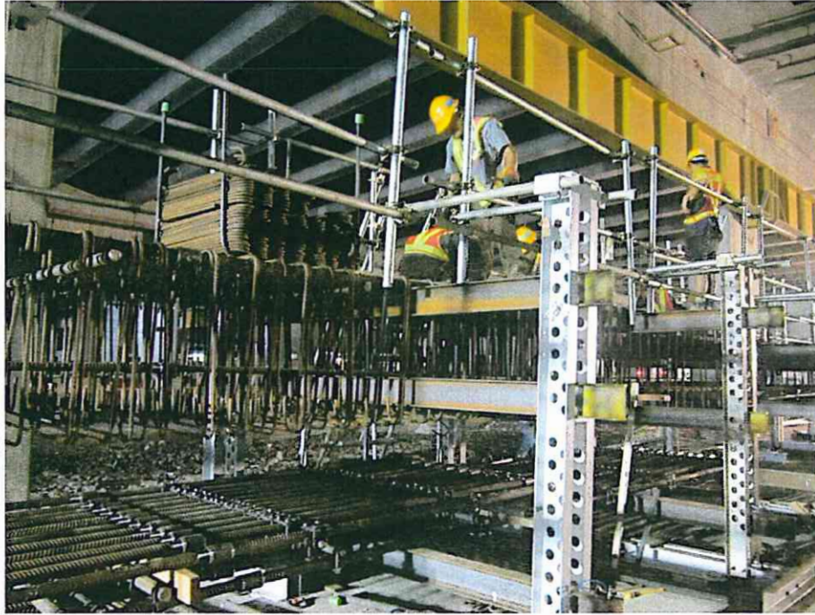
Image 7: fixing of steel cages for panel EM 98 during July 2013 trial
