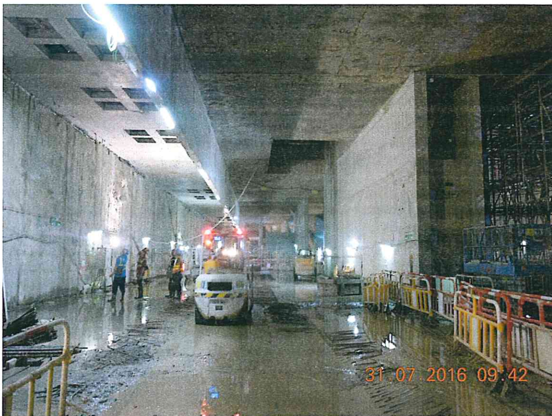
Image 20: general condition of EWL slab soffit after concrete was poured
