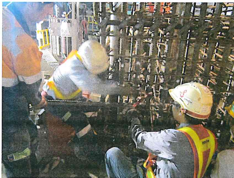
Image 13: splicing works at location of panel EM 98
