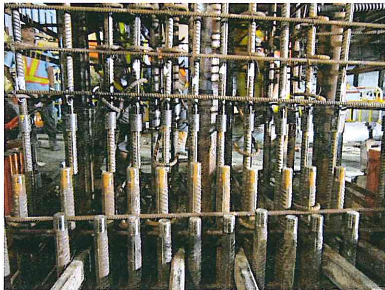
Image 17: completed splicing assemblies of innermost layer for 2 nd and 3 rd steel cages (Note that couplers were properly screwed down but did not have to be flush with each other)
