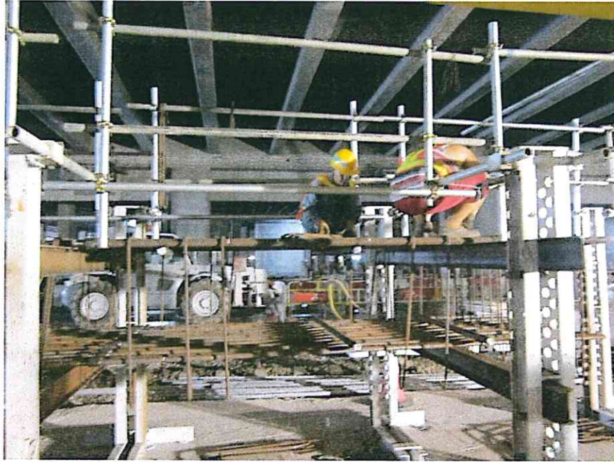
Image 5: fixing of steel cages for panel EM 98 during July 2013 trial
