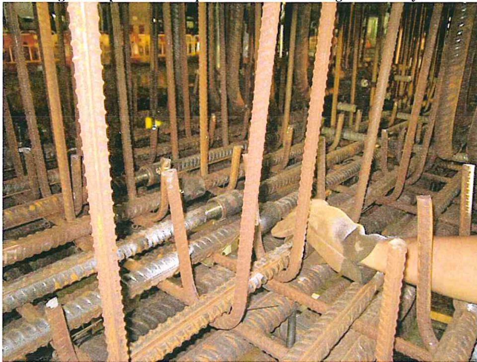
Image 9: inspection of coupler connections during trial in July 2013
