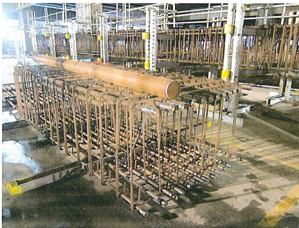
Image 11: disconnection of steel cages for panel EM 98 as part of July 2013 trial
