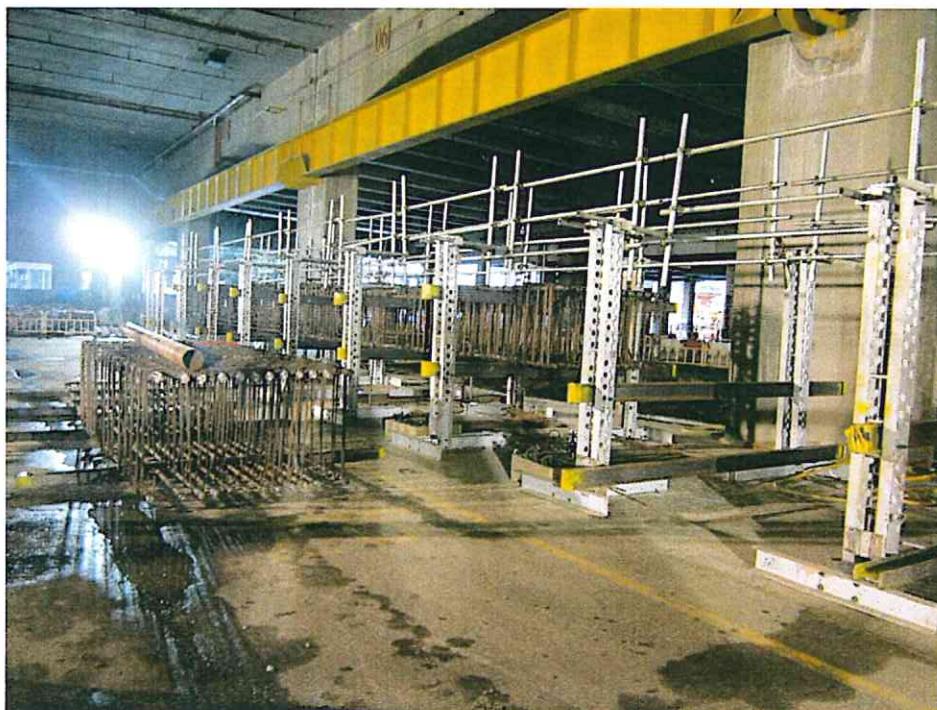
Image 10: disconnection of steel cages for panel EM 98 as part of July 2013 trial
