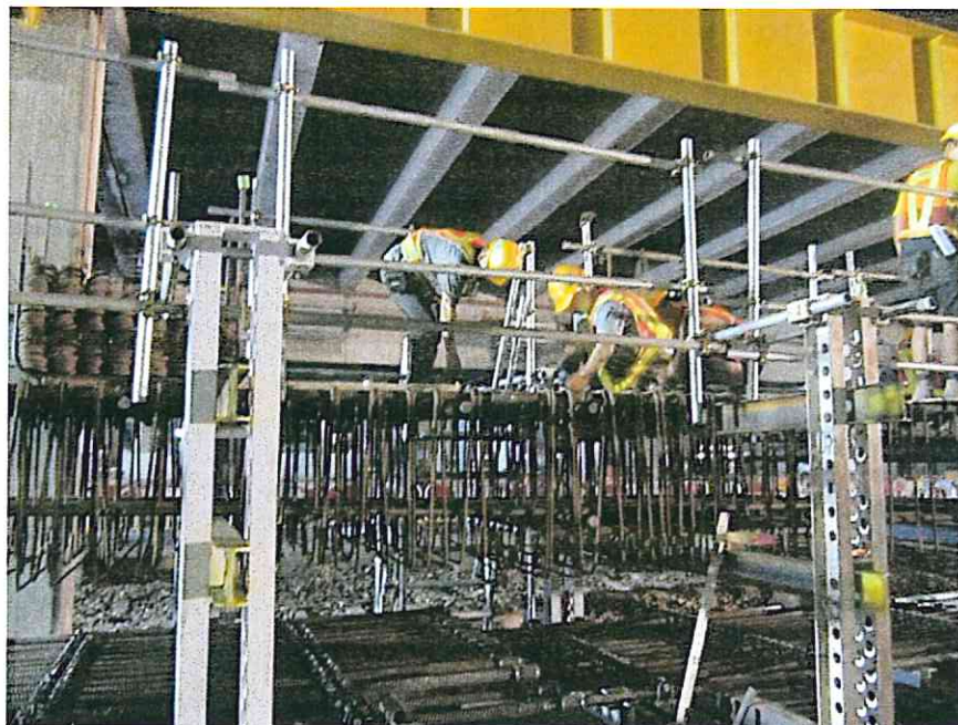
Image 6: fixing of steel cages for panel EM 98 during July 2013 trial
