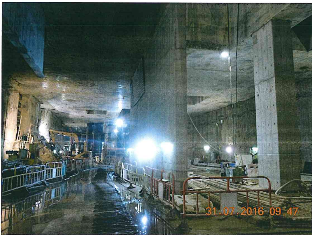
Image 21: general condition of EWL slab soffit after concrete was poured
