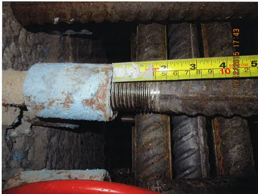
Image 5: measurement of exposed threaded end in Area B-1
