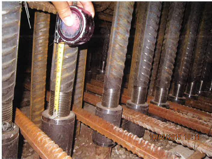
Image 3 – measurement of exposed threading of Type B rebars in diaphragm wall in Area C2-3.
