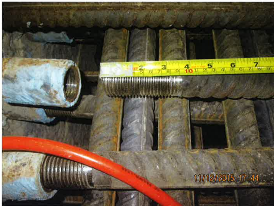
Image 6: measurement of threaded end removed from coupler in Area B-1
